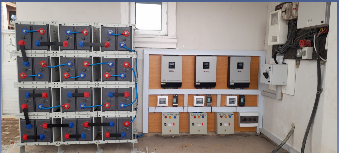
Installation Of 15KW Solar Off-grid System At NAF Valley Estate, Abuja
