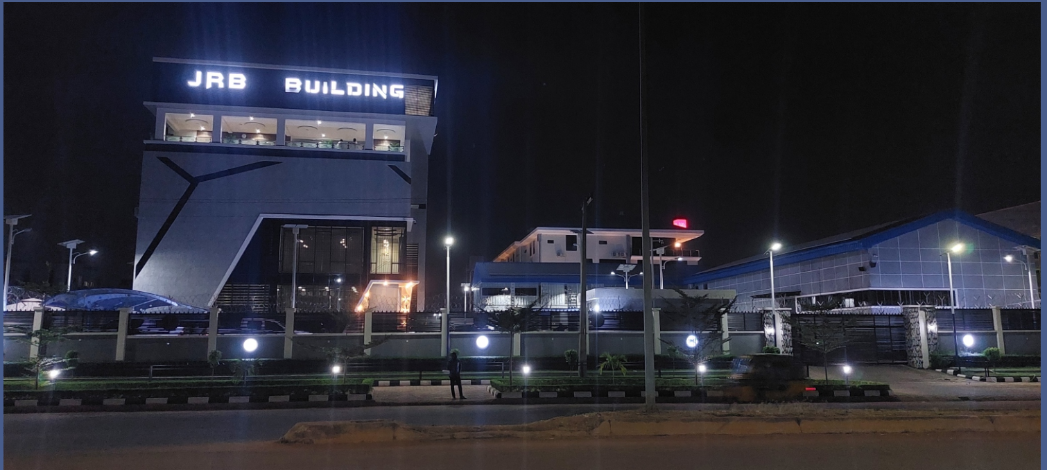
Installation Of 120kw Solar Off-grid System At Our Headquarters In Wuye Abuja
